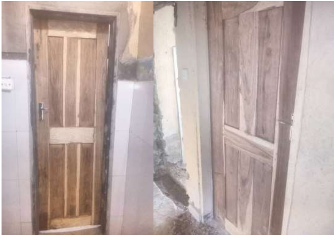
Fig 2: Installation of doors
