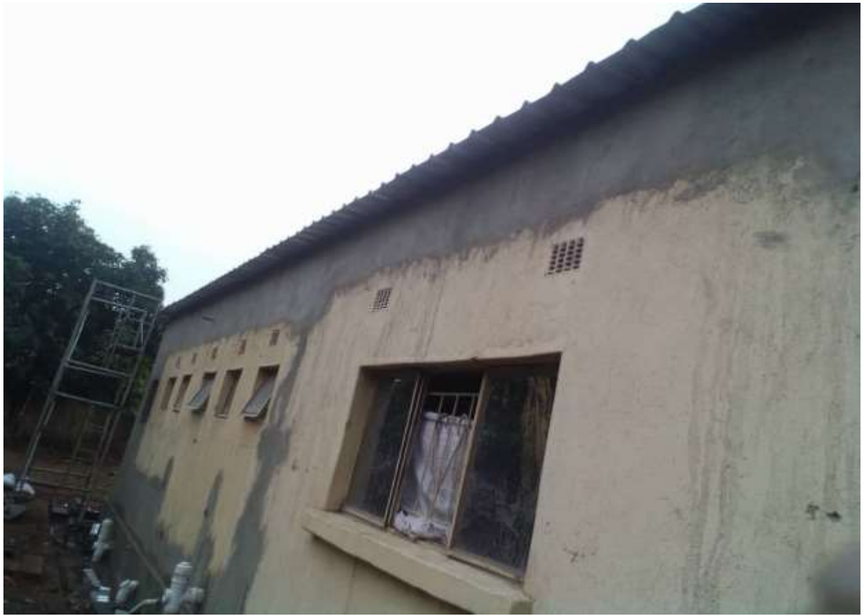
Fig 3: Re-plastering works
